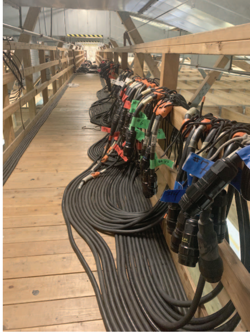
Labeling, color coding, and neatly dressing the cables are key to making a system that works and is maintainable.
