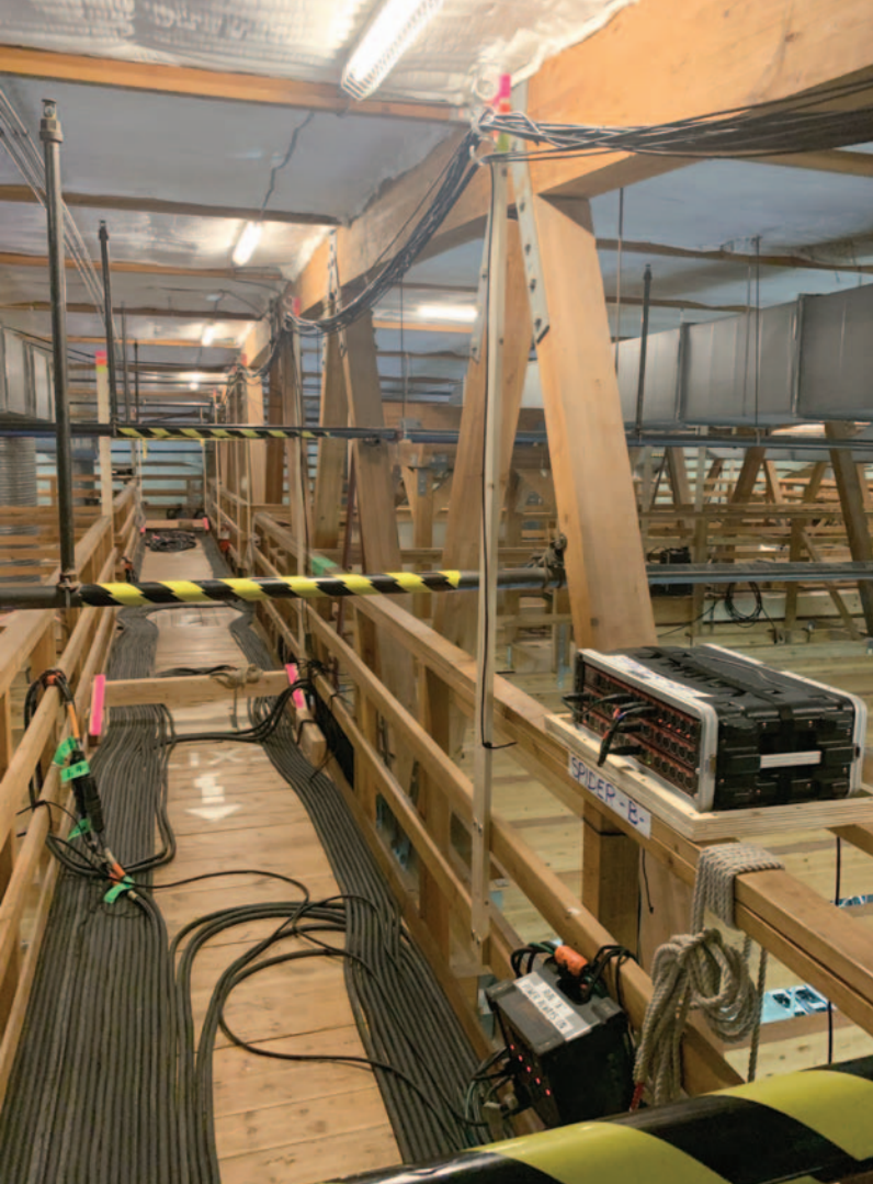
Labeling, color coding, and neatly dressing the cables are key to making a system that works and is maintainable.
